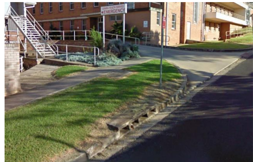
Figure 13 – Kerb converter on Ina Drive - adjacent to emergency vehicle entry. (Source: Google Maps)
